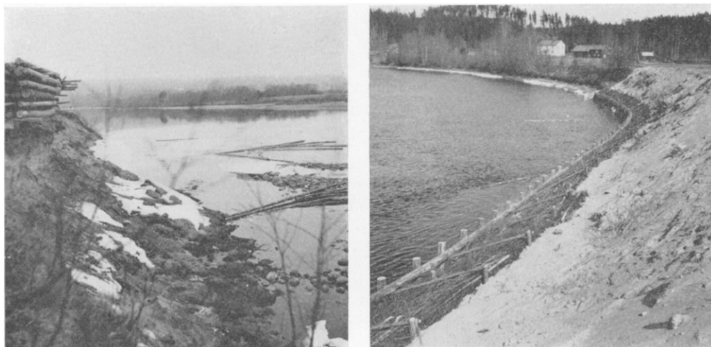
Fig. 38. Left: part of the erosion scarp at Götnäs with the coarse glaciofluvial material projecting above the water level to the right. Right: revetment under erection at Götnäs (April 1954).
